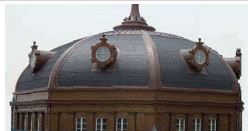
The Roof of one of the Domes (with Japanese Slate)
