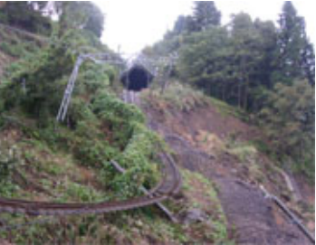
Embankment Collapse (Joetsu Line)
