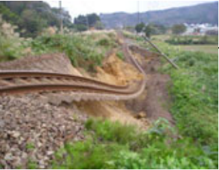
Embankment Collapse (Shin-Etsu Line)
