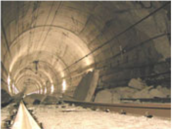
Damaged Tunnel (Shinkansen Uonuma Tunnel)
