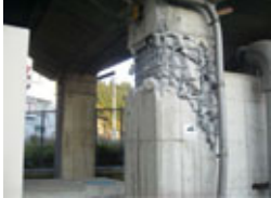
Damaged Bridge (Shinkansen No. 3 Wanazu Bridge)
