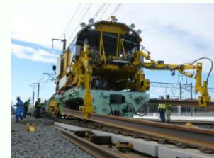
Rail replacement on Tohoku Shinkansen Line
