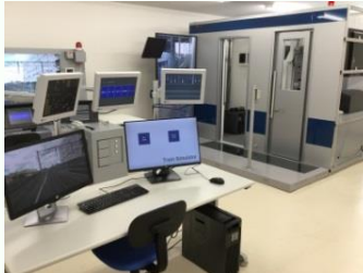
Installation of simulators at drivers & conductors depots
