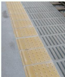
Dot-Braille blocks indicating platform edge
