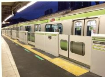
Automatic platform gates installation
