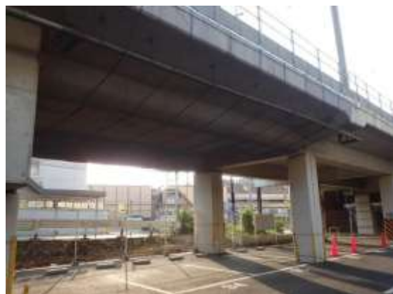
Countermeasure for objects falling from railway viaducts, etc.
