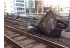
Collapse of electrical pole on Kanda–Akihabara segment of Yamanote Line
