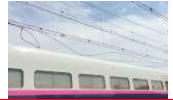
Breakage of overhead wires within Koriyama Station on Tohoku Shinkansen Line
