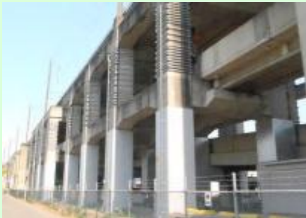
Seismic reinforcement of viaduct columns
