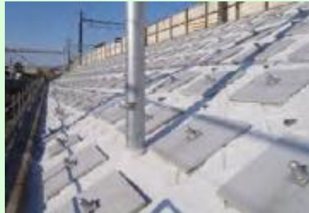
Seismic reinforcement of embankments
