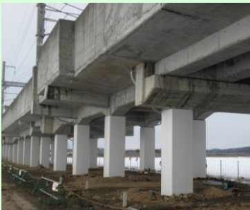
Seismic reinforcement of viaduct columns
