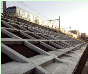
Seismic reinforcement of embankments
