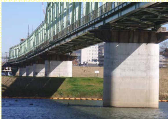
Seismic reinforcement of bridge piers
