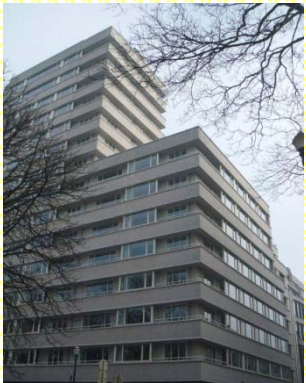
Brussels office (Opened Nov. 1, 2012)
