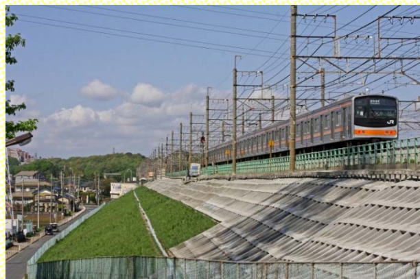
Rainfall disaster prevention (slope reinforcement)
