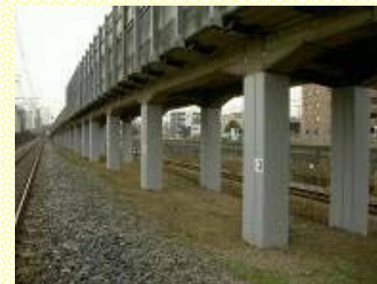
Seismic reinforcement of viaduct columns
