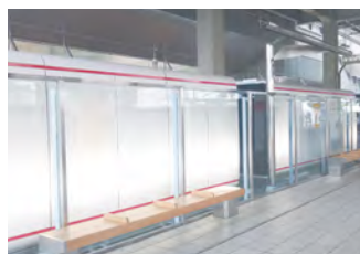
Autonomous hydrogen energy supply system at Musashi-Mizonokuchi Station, a model eco station
