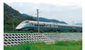
Embankment slope protection (spray-frame work)
