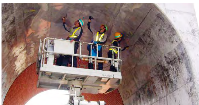
Tunnel inspection training
