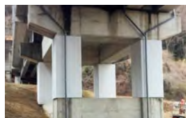
Seismic reinforcement measures (use of steel plate wrapping to reinforce Shinkansen railway viaduct columns)
