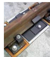
Rail rollover prevention devices
