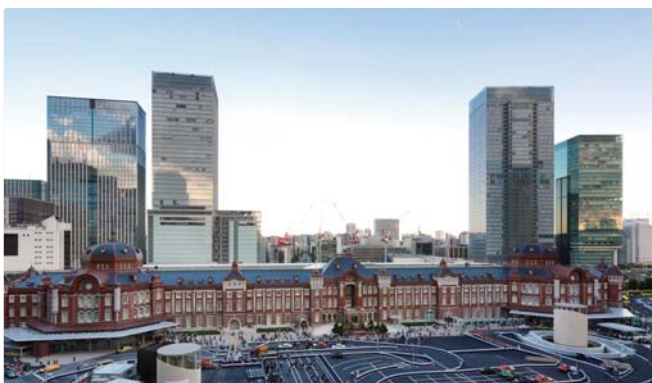
An external view of Tokyo Station City
