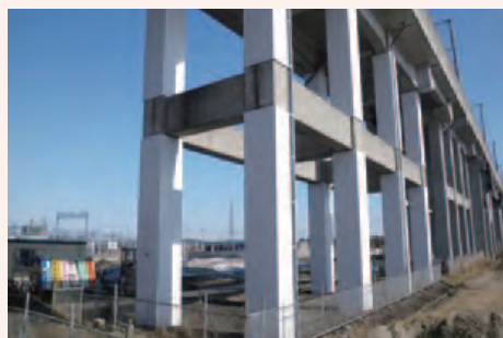
Seismic reinforcement of viaduct columns
