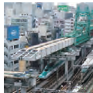
Railway tracks for the Tohoku Through Line under construction
