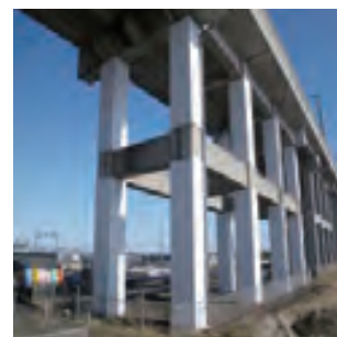
Seismic reinforcement of viaduct columns
