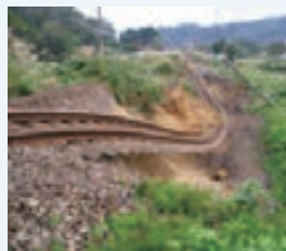
Example of damage
