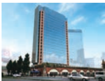
E Kanda Manseibashi Building
