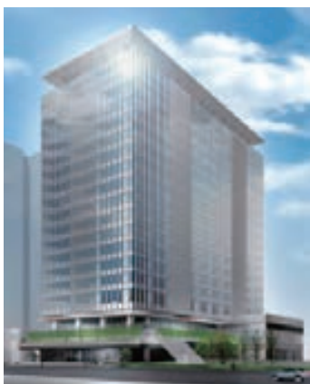
D JR South Shinjuku Building
