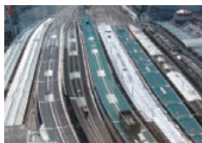
Photovoltaic Panels on Tokyo Station's Tokaido Line Platform (Tracks No. 9 and 10)
