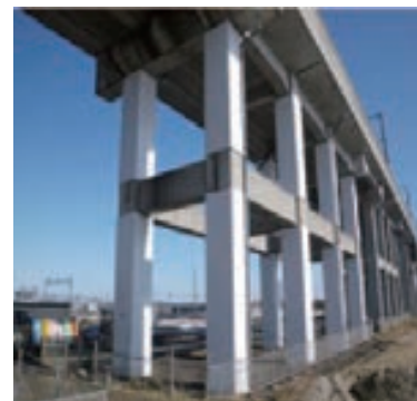
Aseismatic reinforcement of viaduct columns
