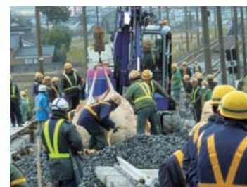
Restoration work on the Joban Line
