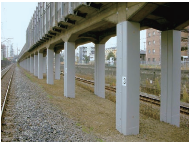
Aseismic reinforcement (Yokosuka Line, between Musashi-Kosugi and Shin-Kawasaki)
