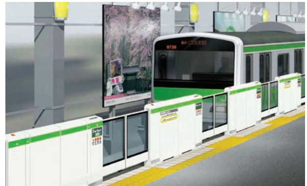
Image of automatic platform gates
