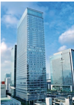
GranTokyo South Tower
