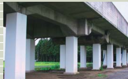
Reinforcement of supports for elevated Shinkansen tracks
