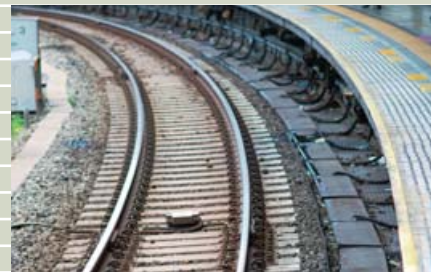
Sensor mat for halting train movement when a passenger has fallen from a platform onto the track area.
