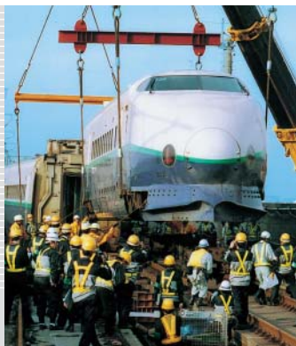
A scene of restoration work
