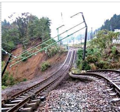
Joetsu line between Echigo Kawaguchi and Ojiya after the Earthquake
