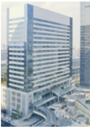
JR Shinagawa East Building
