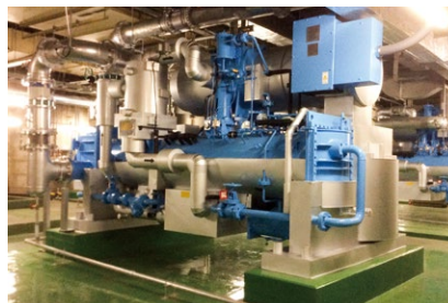
High-efficiency turbo refrigeration and air conditioning units after facility upgrading
