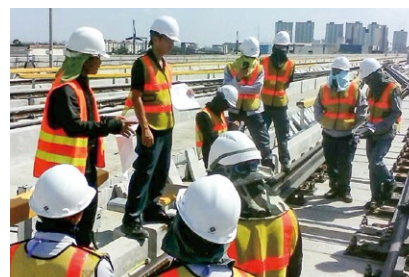
Maintenance of track for vehicle
