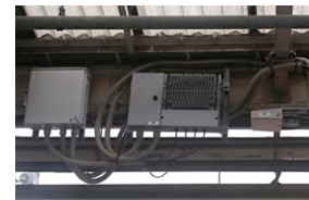
Improvement of a WiMAX base station
