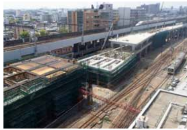
Railway overpass construction project near Niigata Station on the Shin-etsu Main Line
