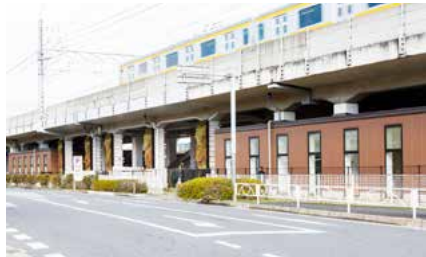
Nursery school under elevated railway tracks (Ichikawa Doronko Nursery)
