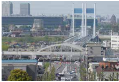
Railway overpass construction project near Inagi-Naganuma Station on the Nambu Line
