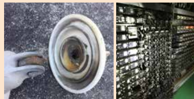
March 15, 2016 Transport disrupted by breakdown of electrical equipment at Kagohara station on the Takasaki line
