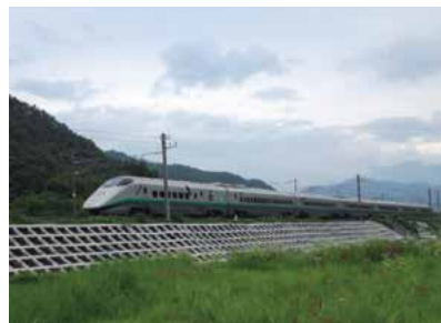
Embankment slope protection (spray frame work)
