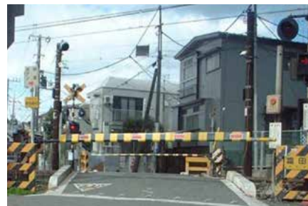
A large crossing gate
