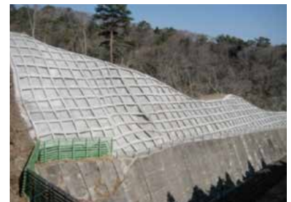
Natural slope protection (spray frame work)
