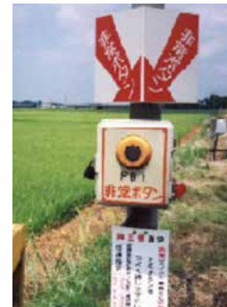
Level crossing alarm system
