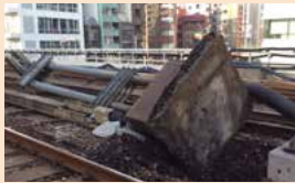
April 12, 2015 Electric post collapsed between Kanda and Akihabara on the Yamanote line (serious incident)
