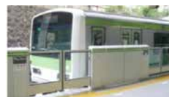
Automatic platform doors
