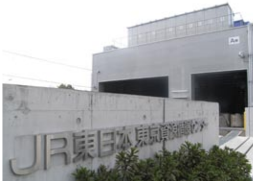
JR East Tokyo Materials Recycling Center
