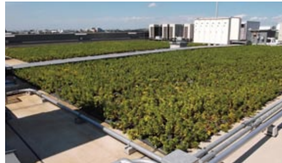
Rooftop greening at the Chiba branch building
