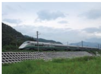
Embankment slope protection (spray frame work)
