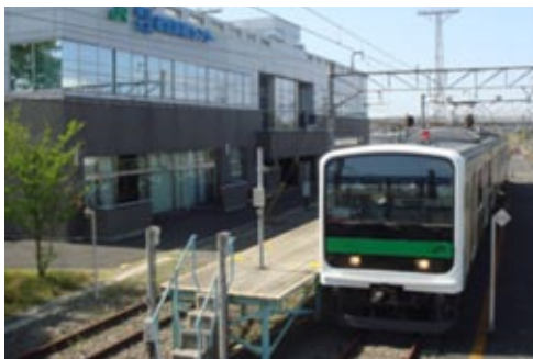
Training train and training tracks at Tokyo/Omiya General Training Center
