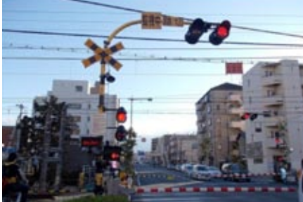
A crossing warning device located in a higher position for better visibility
