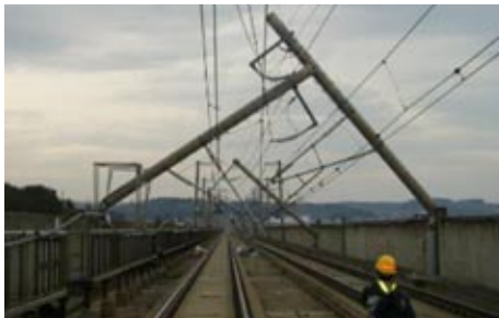
[Reinforcement of electric poles and installation of a beam to make it a gate shape]
