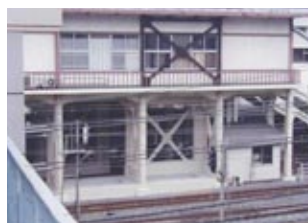
Reinforcement by steel frame braces
