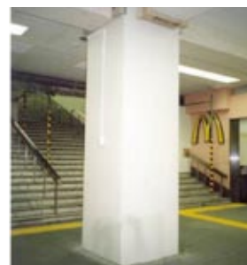
Reinforcement of columns by steel plate wrapping
