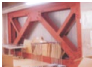
Reinforcement by steel frame braces
