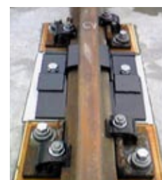
Rail rollover prevention devices
