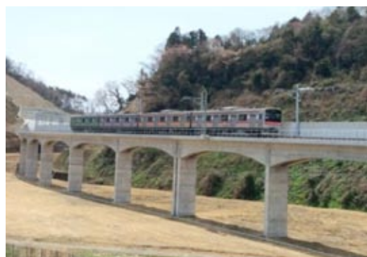
Senseki Line (between Nobiru and Rikuzenono)
