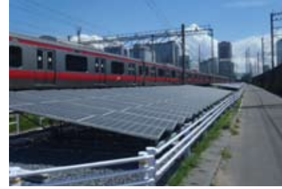
Solar panels installed at Keiyo Rolling Stock Center
