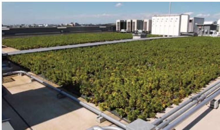
Rooftop greenery at the Chiba branch building
