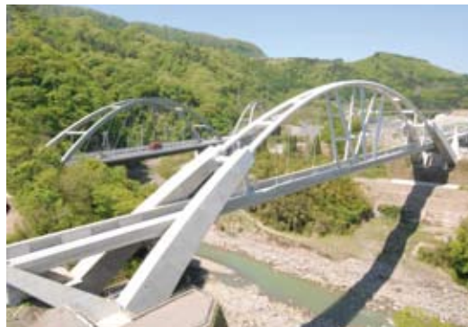
Agatsumagawa Bridge No. 3
