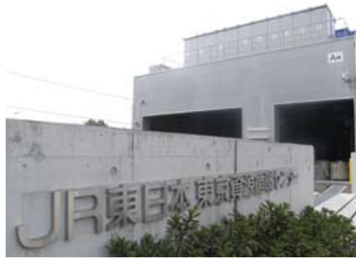
JR East Tokyo Materials Recycling Center
