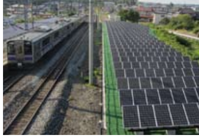
Solar panels at Hiraizumi Station
