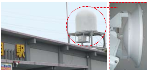
Doppler radar installed on the roof of Amarume Station on the Uetsu Line
