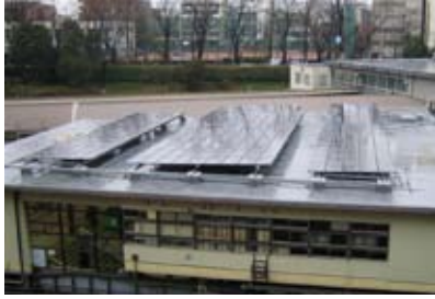
Solar panels on the main building at the Akasaka Exit of Yotsuya Station
