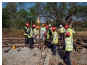
Track maintenance in Myanmar (PC sleeper replacement)
