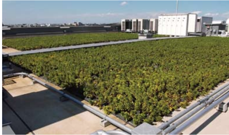
Rooftop greenery at Chiba branch building
