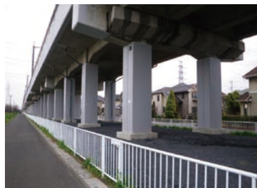
Examples of seismic reinforcement
