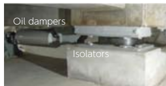
Installed vibration control system
