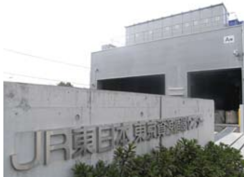
JR East Tokyo Materials Recycling Center
