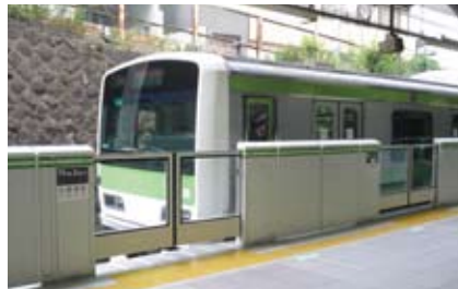
Automatic platform gates on the Yamanote Line
