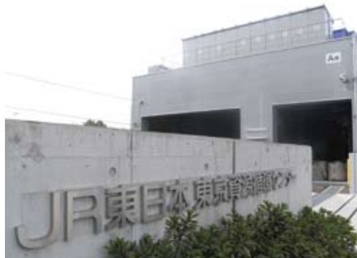
JR East Tokyo Materials Recycling Center
