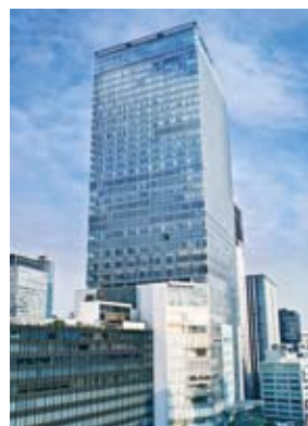
Gran Tokyo North Tower, recognized as a top-level establishment
