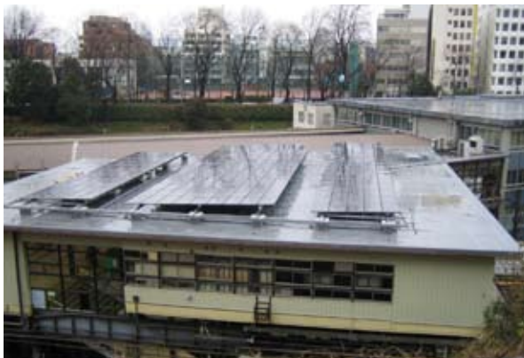
Solar panels on the main building at the Akasaka Exit of Yotsuya Station
