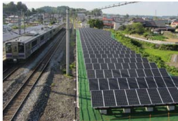
Solar panels at Hiraizumi Station
