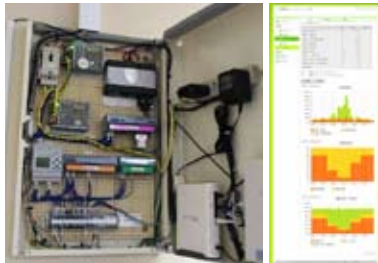
Visualizing energy savings by installing an artificial intelligence panel, increasing energy management efficiency
