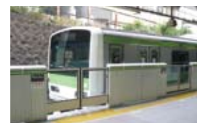
Automatic platform gates on the Yamanote Line
