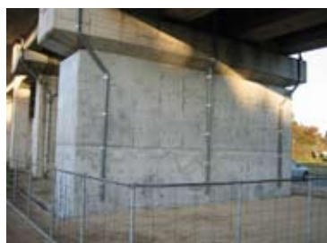
Examples of seismic reinforcement
