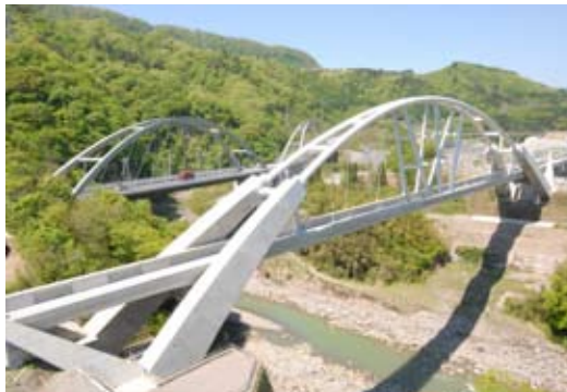
Agatsumagawa Bridge No. 3
