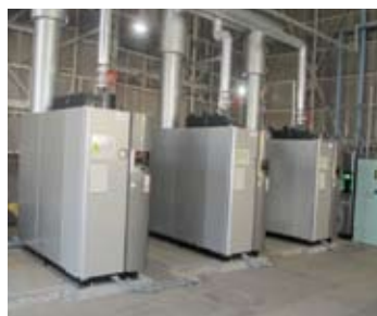
CO 2 reduction by changing fuels for once-through boilers
