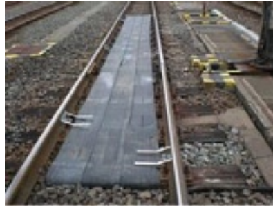
Snow-melting equipment using hot water mats
