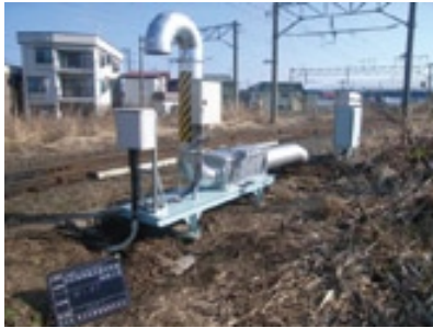
Snow-melting equipment using hot air with gas
