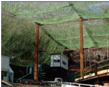
Reducing visual impact using camouflage netting
