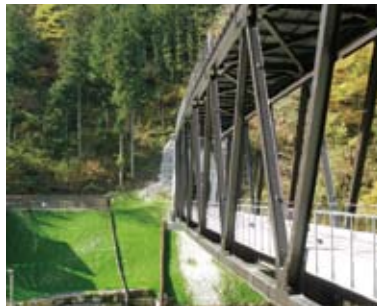
Sprigs planted at Shiroiwasawa Bridge
