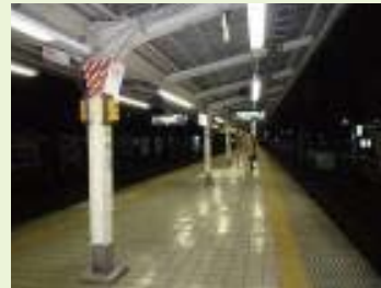
After: Intensity is even throughout the platform after changing the layout of lighting apparatus
