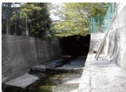
Routing tunnel groundwater to the Tachiaigawa River
