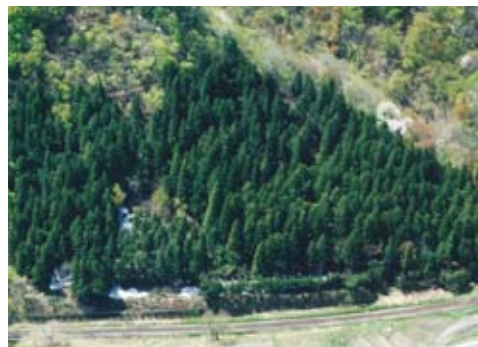
Tenoko No.6 railway forest on the Yonesaka Line (forest to protect against snowslides)
