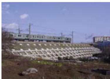
Concrete lattice frame protection work
