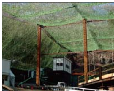
Reducing visual impact using camouflage netting
