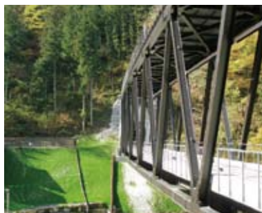
Sprigs planted at Shiroiwasawa Bridge
