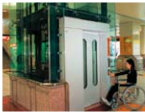
Overcoming differences in levels by installing elevators
