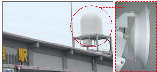
Doppler radar installed on the roof of Amarume Station on the Uetsu Line Doppler radar body
