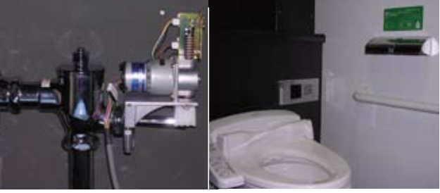
Automatic water flow controller for toilets (BT-Crab)—reduces toilet water consumption by 50%
