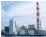
At Kawasaki thermal station kerosene was replaced with natural gas to run No. 3 generation unit in June 2006.
