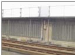
Installing sound-absorbing panels
