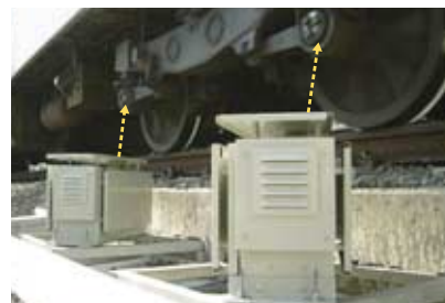
Axle box temperature detection equipment [axle boxes are indicated by the yellow arrows]
