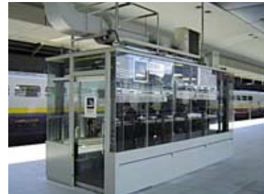
Air-purifier-equipped smoking rooms on Shinkansen station platform
