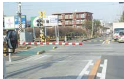
A red and white large crossing gate, to improve visibility and deter careless crossing of railway tracks
