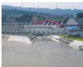
The disaster-damaged Shinanogawa hydropower plant has been restored.
