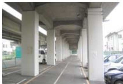
Reinforcement of seismic resistance of Shinkansen viaduct support columns is being carried out as planned.
