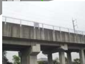
Raising the height of soundproof walls
