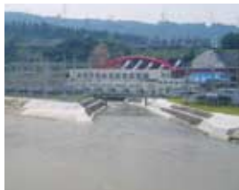
The disaster-damaged Shinanogawa hydropower plant has been restored.
