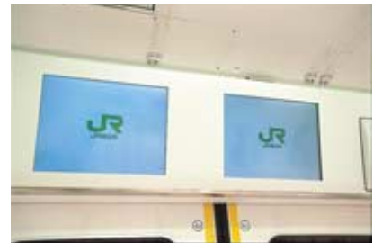
The LC display above the door provides information about operations and transfers as well as news and weather forecasts
