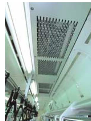
Air-purifiers installed for the first time on commuter-type railcars
