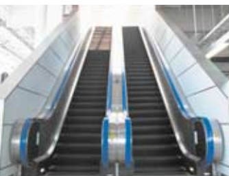
Up and down escalators
