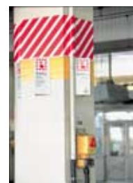
An emergency stop button, one of our systems for stopping trains in emergencies, installed on a post along a platform
