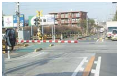
A red and white large crossing gate, to improve visibility and deter careless crossing of railway tracks
