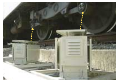
Axle box temperature detection equipment [axle boxes are indicated by the yellow arrows]
