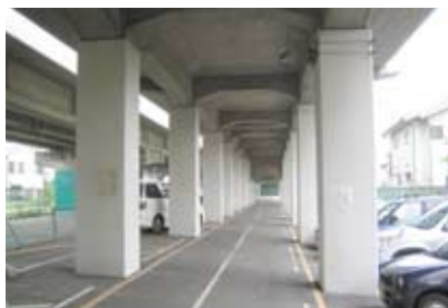
Reinforcement of seismic resistance of Shinkansen viaduct support columns is being carried out as planned.
