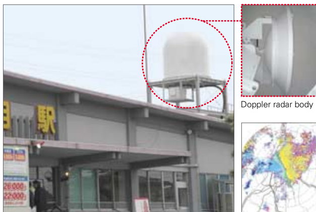
Doppler radar installed on the roof of Amarume Station on the Uetsu Line
