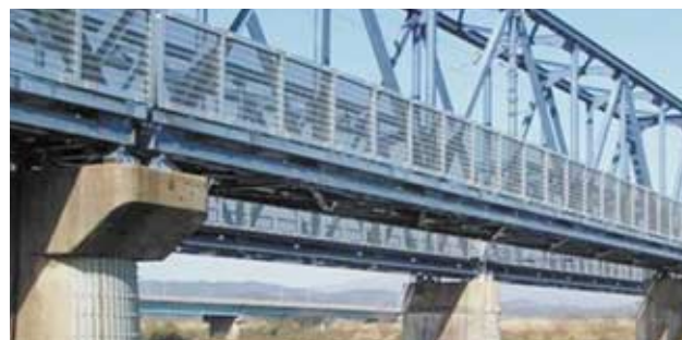
Windbreak fence installed at the No.2 Mogamigawa Bridge
